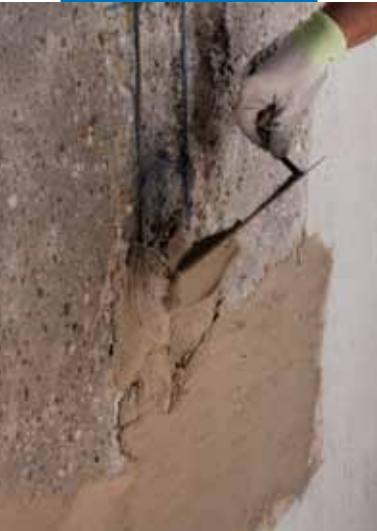
Application of Planitop Smooth & Repair by trowel
